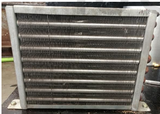
Fig. 2 Conventional Air Cooled condenser
